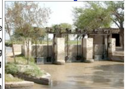
Regulator gates at canals control the flow of irrigation water
